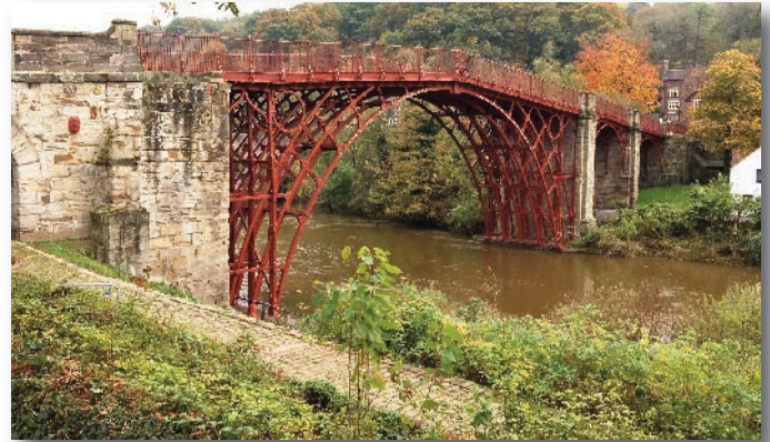
Built in 1779, this bridge that crosses the Severn River in Shropshire, is the oldest cast iron bridge in the world.
