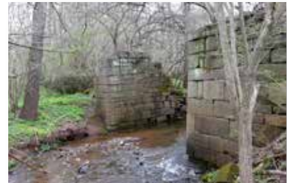
Seltzer's Aqueduct supports on the Girard Canal
